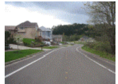
New roadway standards in practice
