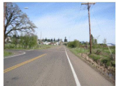
Bellfountain Road – Urban Collector
